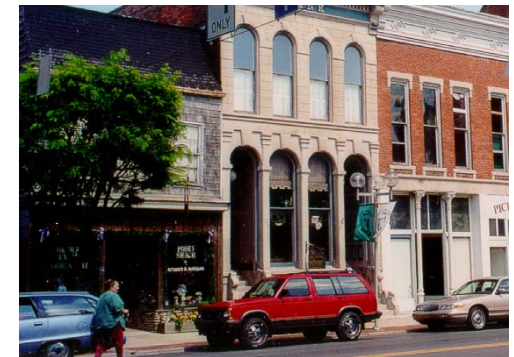
On street parking should be provided wherever possible to allow convenient access to local business and amenities.
